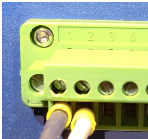
Figure 3: Power-supply of the laser
